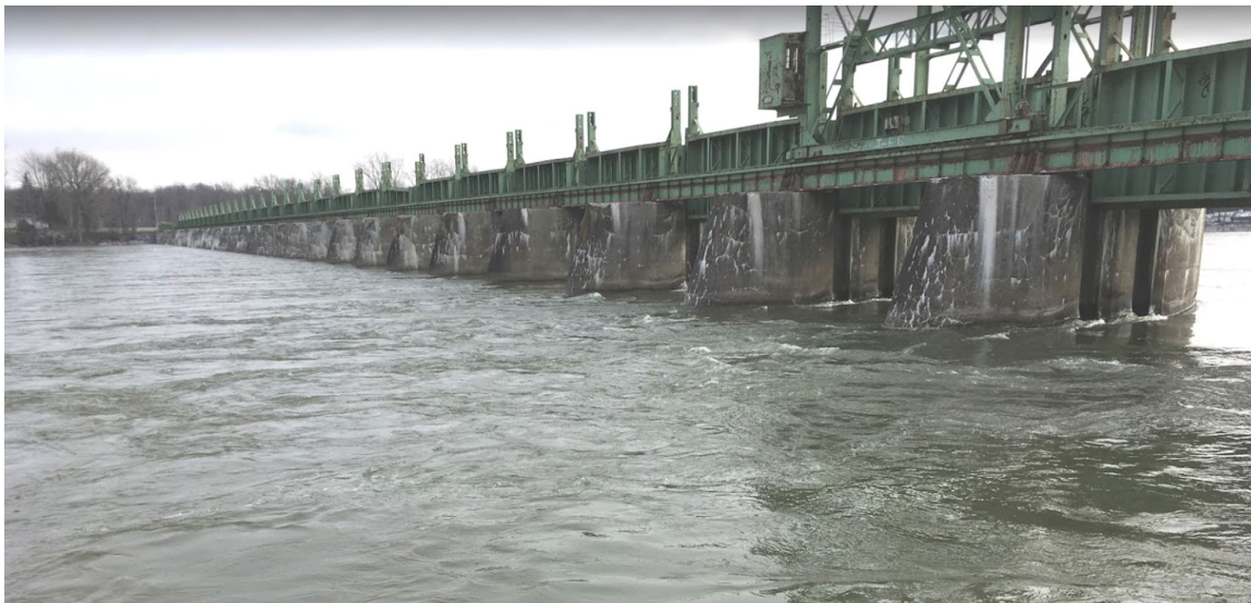
Figure 4-1 | Fryer Island Dam ( https://www.pc.gc.ca/en/lhn-nhs/qc/chambly/culture/ingenierie-engineering/barrage-fryer-dam )
