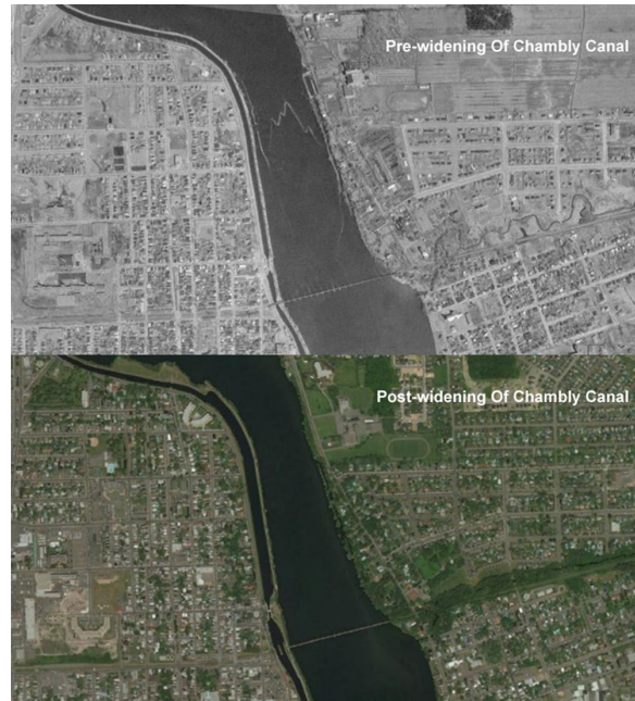
Figure 4-4 | Chambly Canal widening
